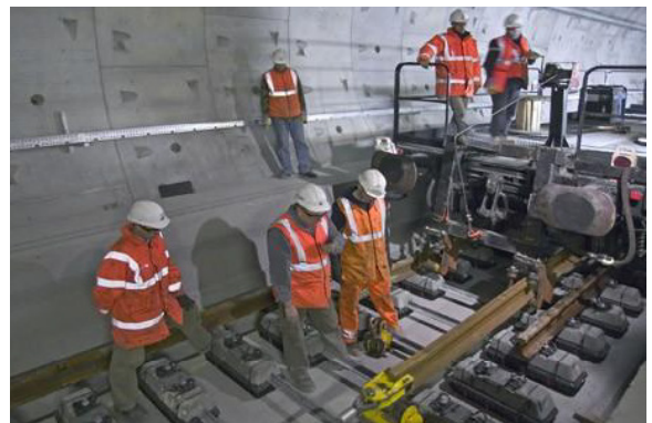
Adding the rails onto the sleepers
