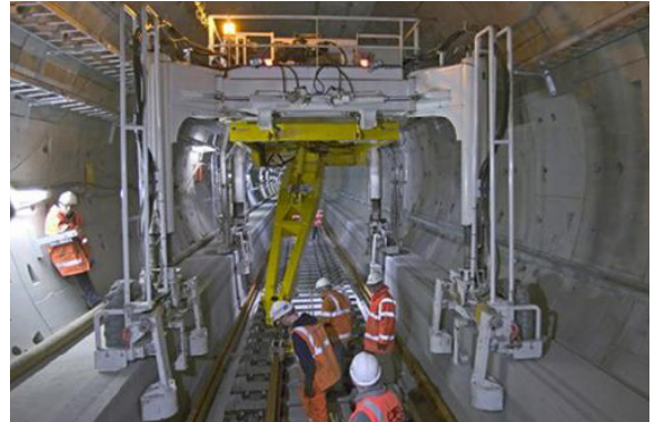
Sleepers installed in bails of 10
