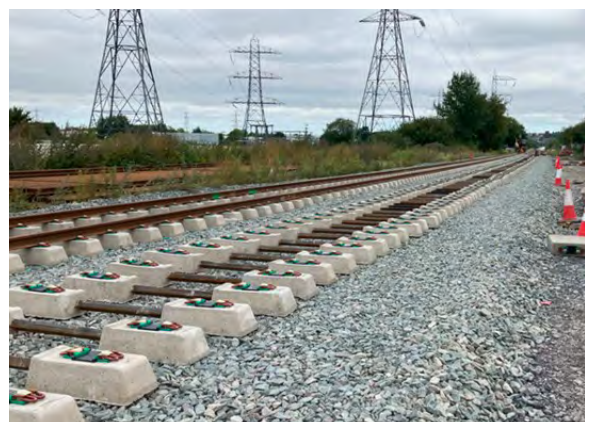
VAX U21 Sleepers being installed on West Midlands Metro line extension
