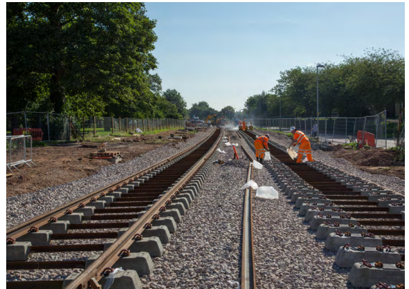
VAX U21 sleepers used for ballasted track
